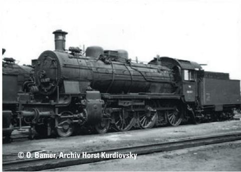
**Prototype:** Austrian Federal Railways (ÖBB) class 638 passenger locomotive. Former Prussian class P 8. Boiler with 3 domes and without smoke deflectors. Four-axle box-style tender, pilot truck with solid wheels.
